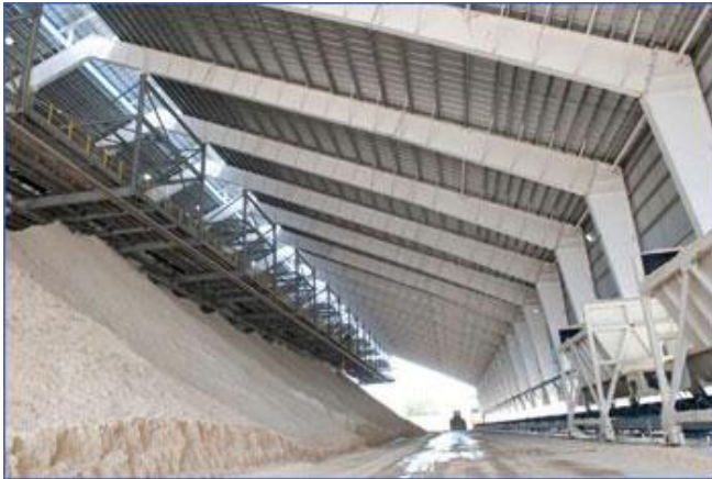
Figure 2. Gypsum storage hangar
